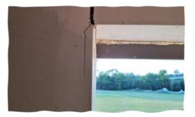
The photographs above show the Playing Field Pavilion has large cracks across the floor and down the front and back wall. These cracks are growing longer and wider and the roof is unstable.
