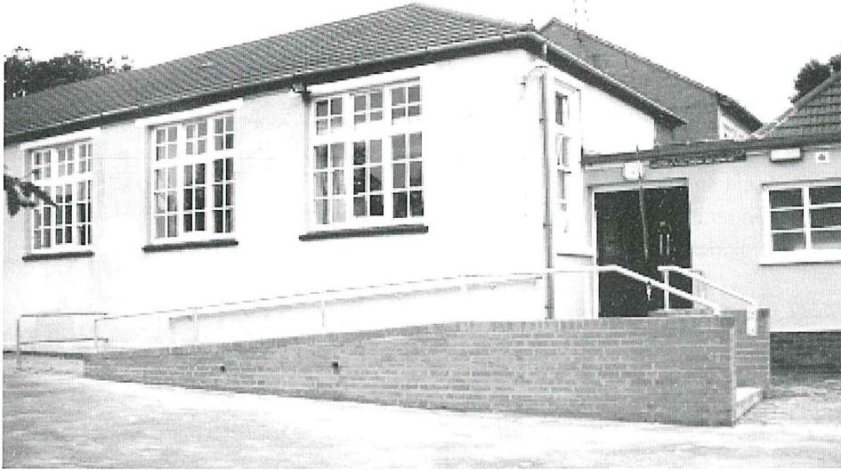
Outside of the Hall showing new access ramp for wheelchair users
